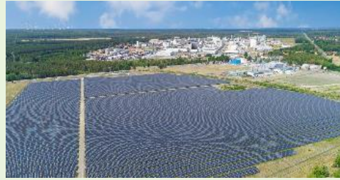
On-site solar park Schwarzheide, Germany
