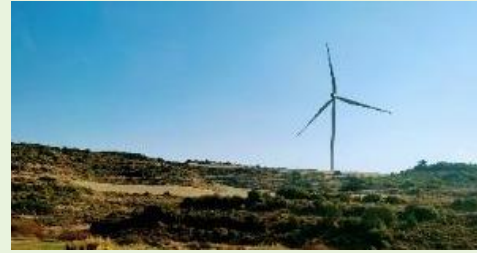
25 years onshore wind power from Spain
